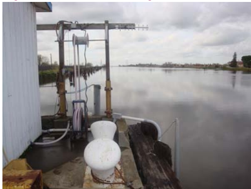
Figure 3 - Burns Cutoff Gage Station
