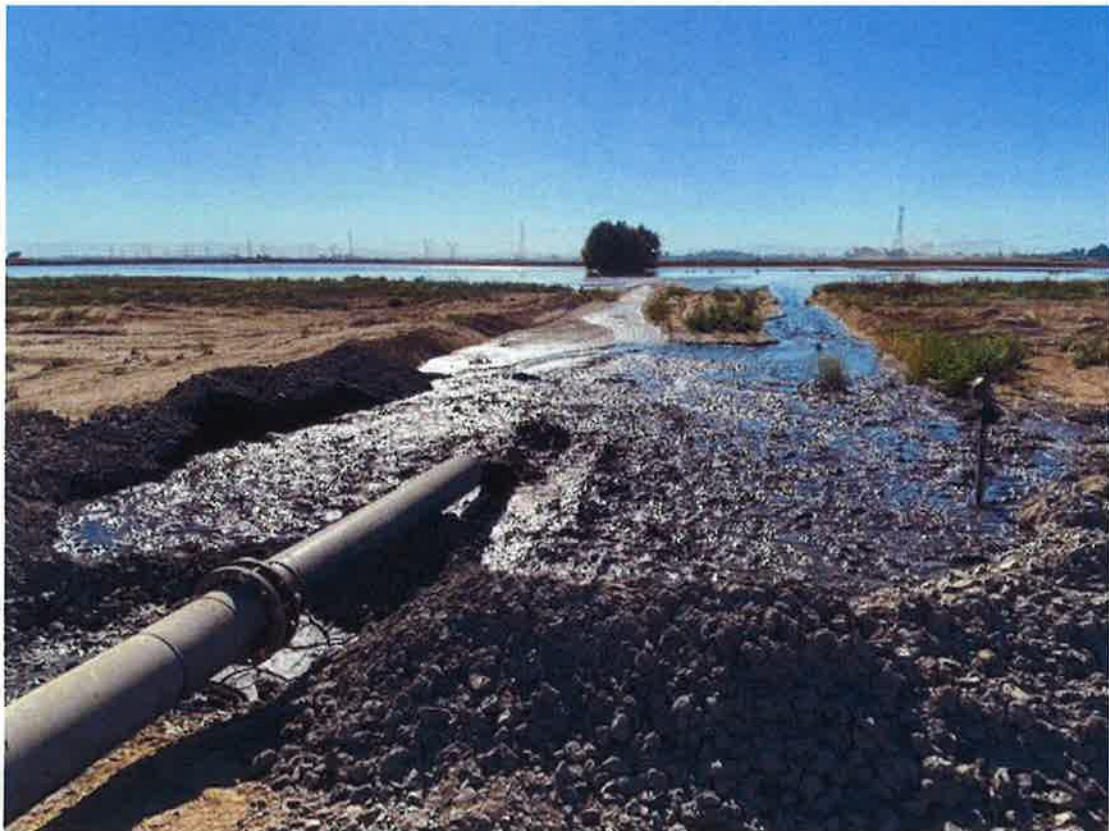
Dredge Discharge At Lower Roberts Sediment Pond
