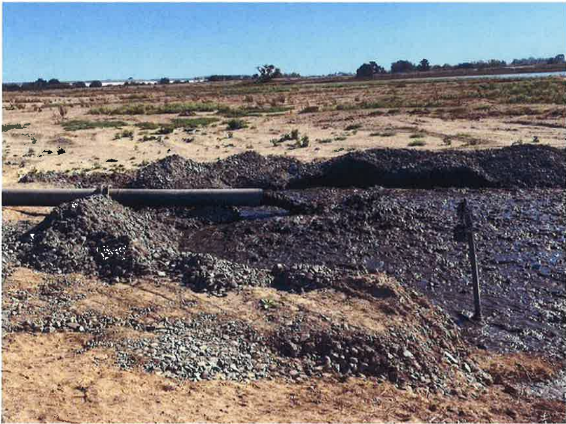
Dredge Discharge At Lower Roberts Sediment Pond
