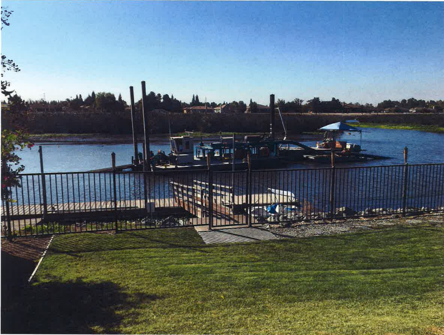
Fourteen Mile Slough Dredging Operations
