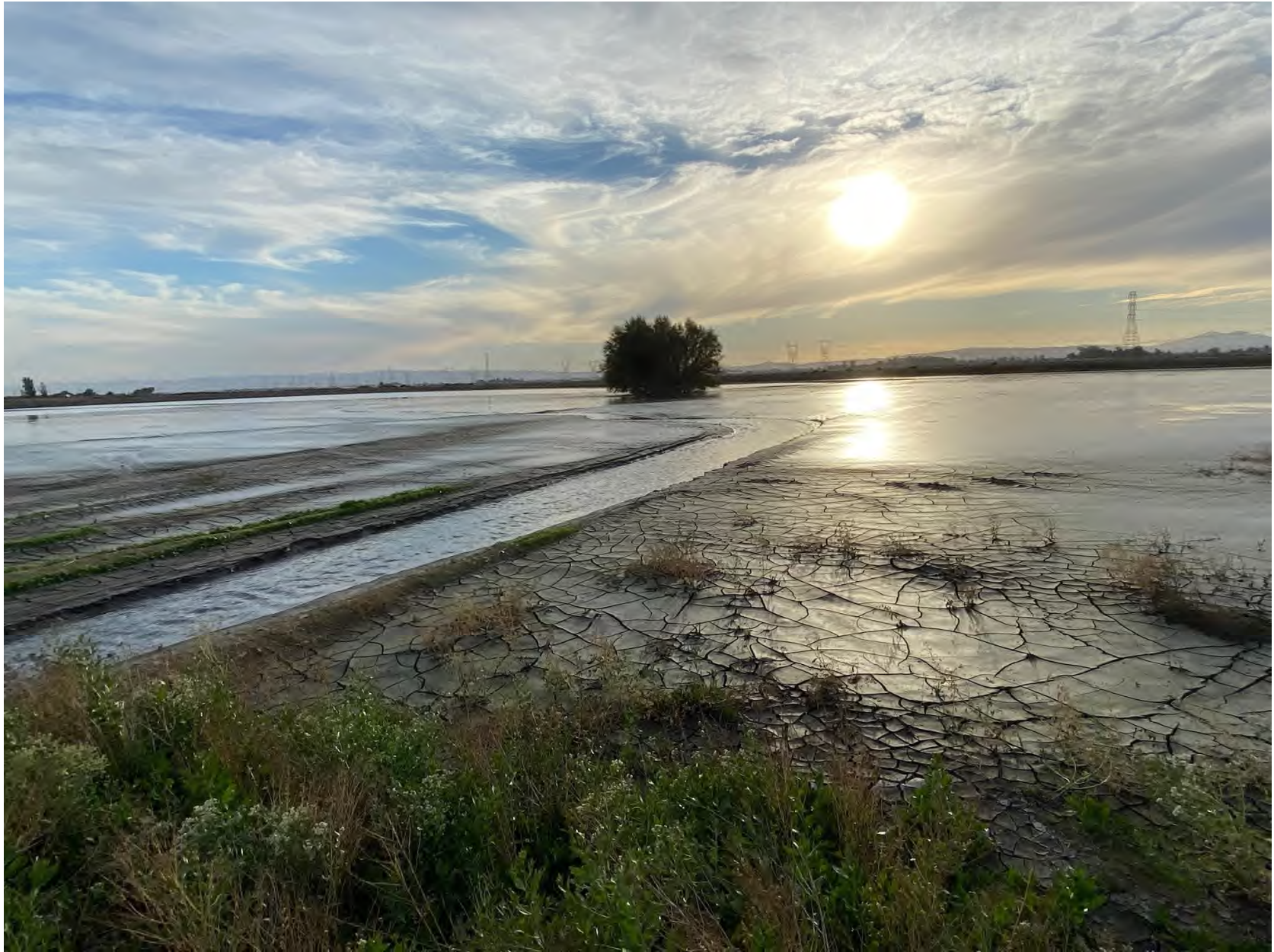
Sediment Storage Pond
