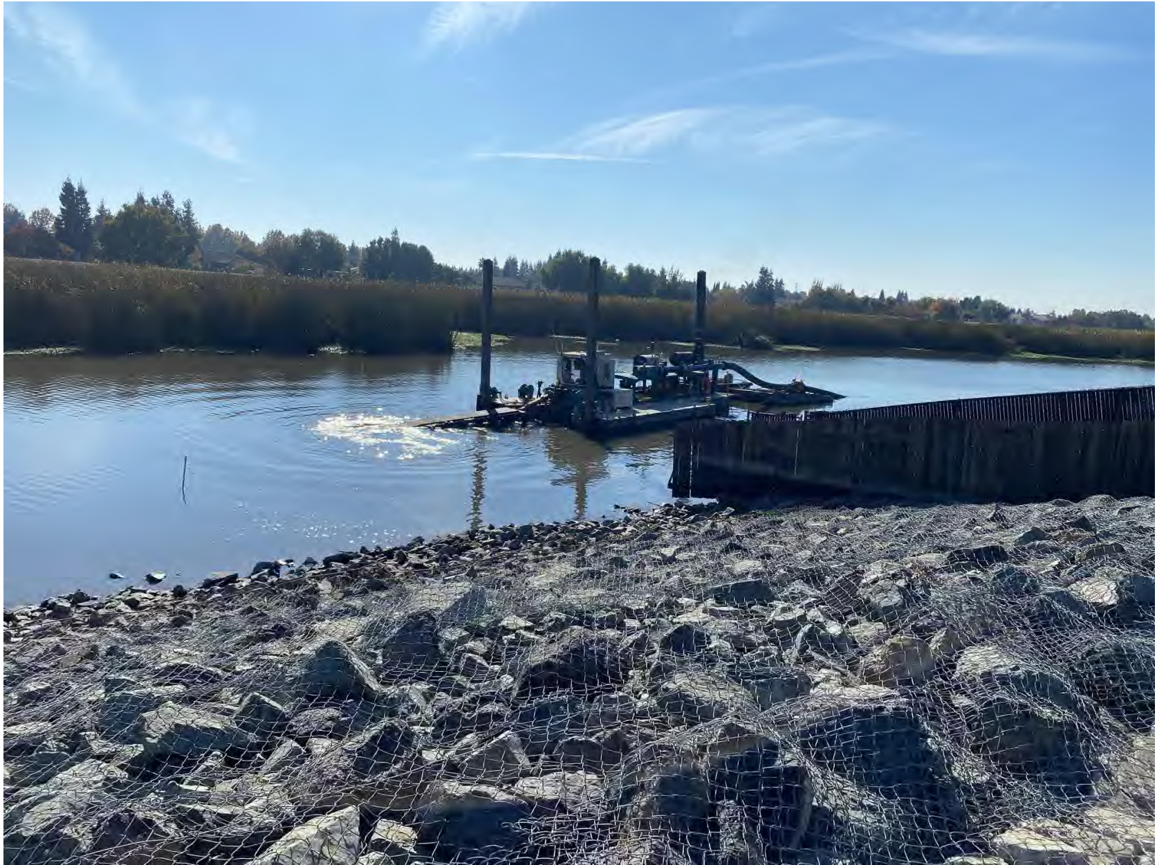
Dredging near Grupe Park
