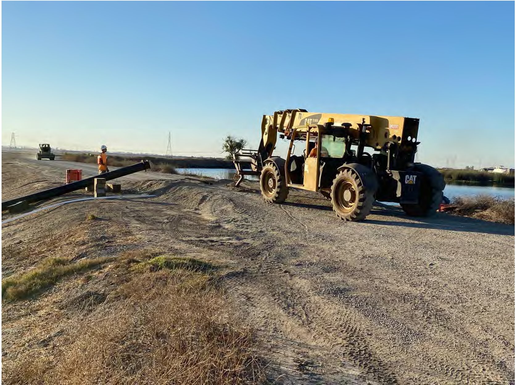
Demobilization of sediment transport pipe underway
