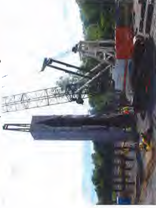
Pile Driver without Noise Reduction Equipment Source: Carpenters Training Institute
