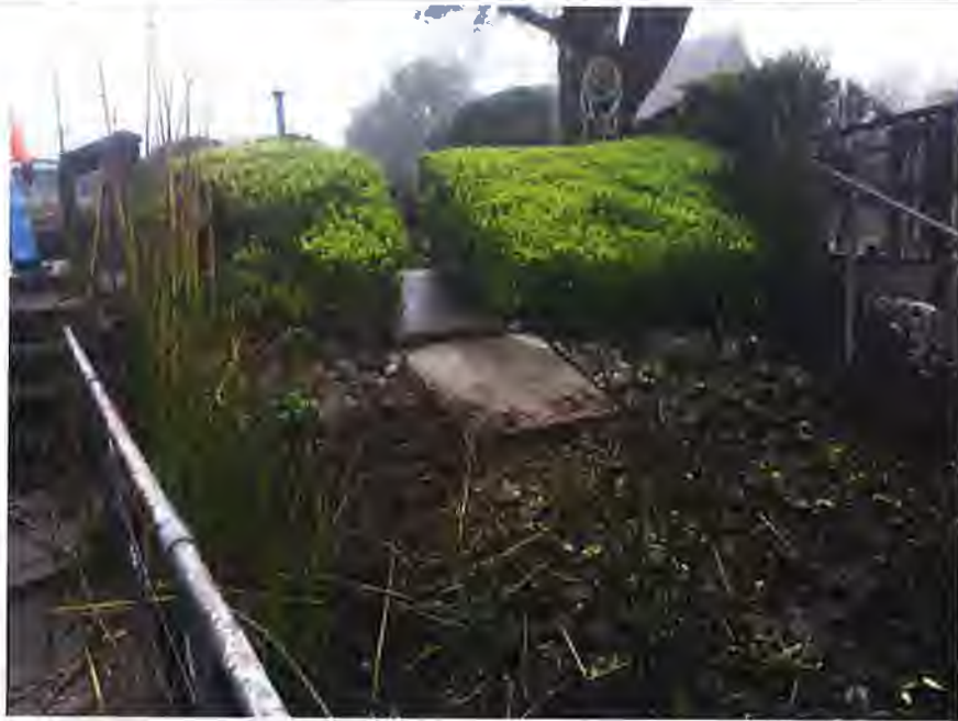
The southeast waterside levee slope.
