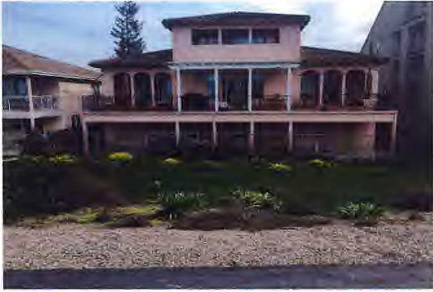
Before Vegetation Removal
