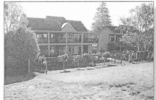
Example of well-trimmed bushes allowing levee inspection.
