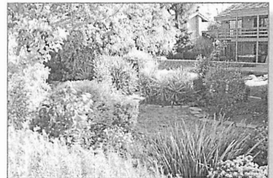
Example of poor vision of levee toe that could hide levee damage.
