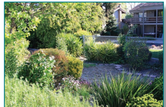
Example of poor vision of levee toe that could hide levee damage.
