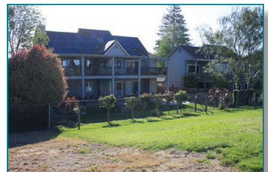
Example of well-trimmed bushes allowing levee inspection.
