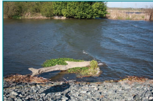
Example of floating debris brought in by high water and ultimately removed by Joe to avoid damaging the rock slopes.
