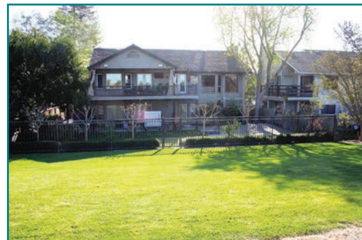
Example of well-maintained view of levee toe.
