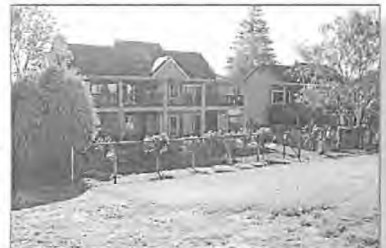
Example of well-trimmed bushes allowing levee inspection.
