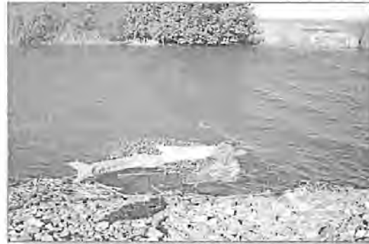
Example of floating debris brought in by high water and ultimately removed by Joe to avoid damaging the rock slopes.
