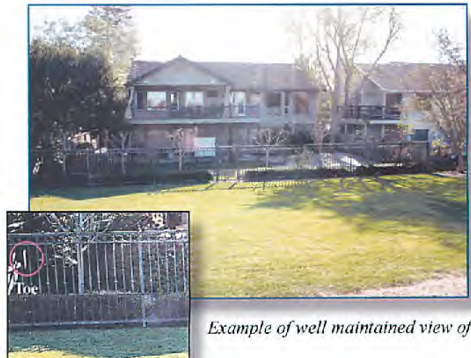
Example of poor vision of toe that could hide levee damage
