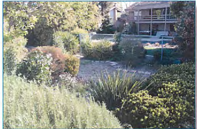
Example of poor vision of toe that could hide levee damage
