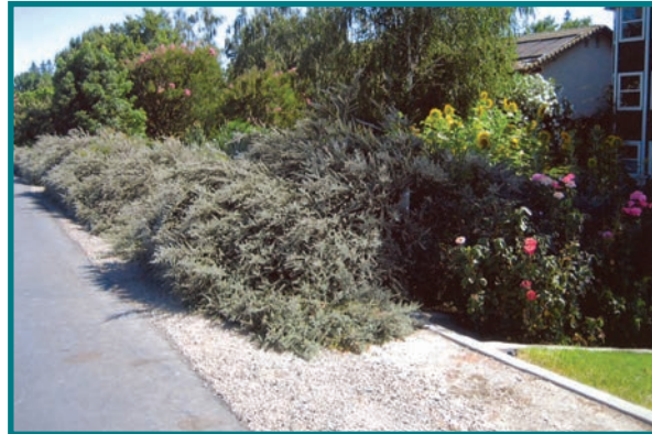
Non-compliant intrusion of vegetation on the levees.
