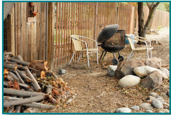
Inappropriate use of levee for storage
