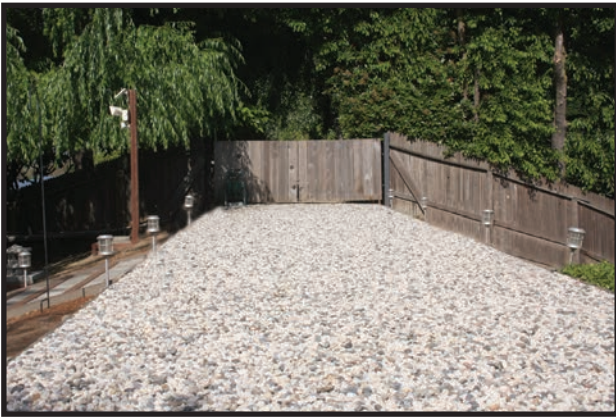
Good. Clear gate access to the levee.
